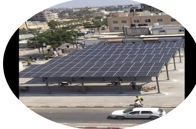
Khan Yonis - Construction of Municipal Main Garage
