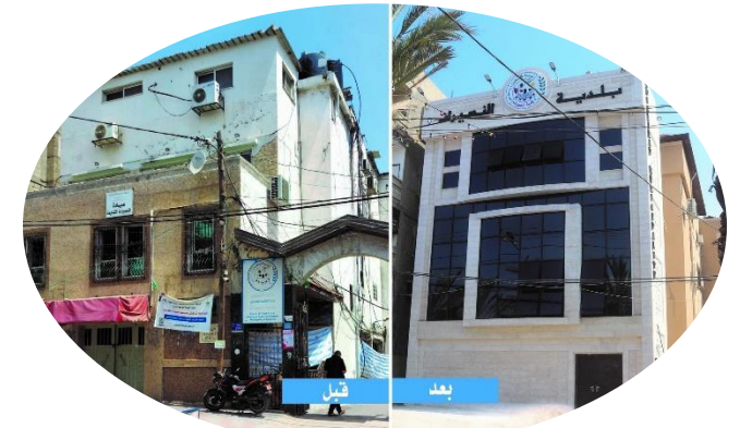
Al Nusseirat - Rehabilitating of Municipality building
