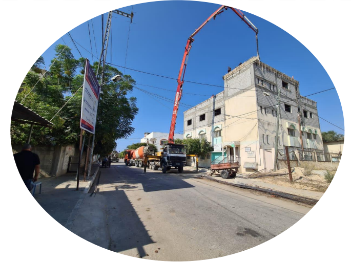
AL Mussader - Construction of 2nd floor
