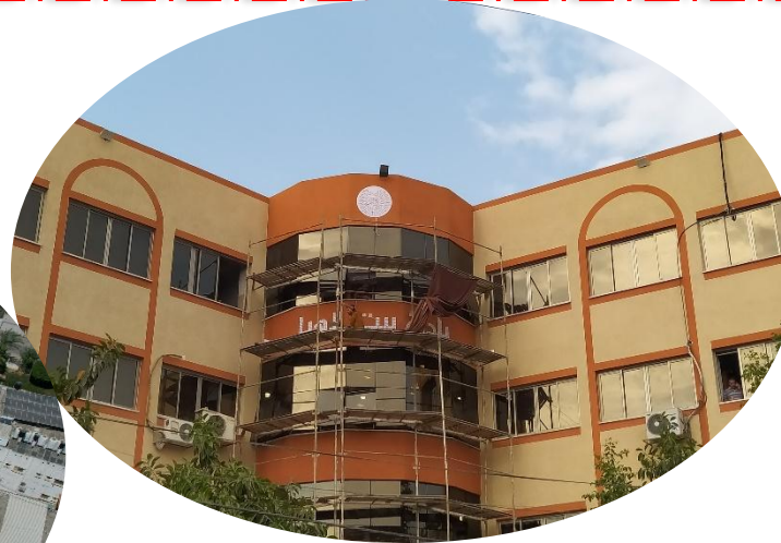
Beit Lahia - Maintenance the main building
